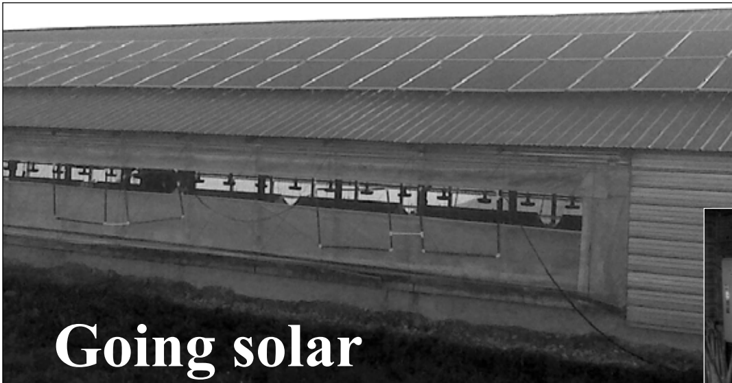
LEFT: The Van Metre poultry house with solar panels on the southside roof.
